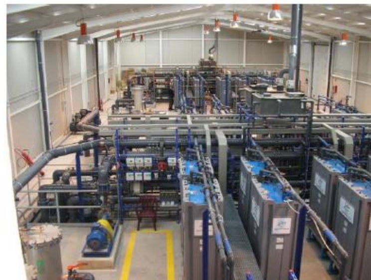
Figure 2: Installed EDR Systems
