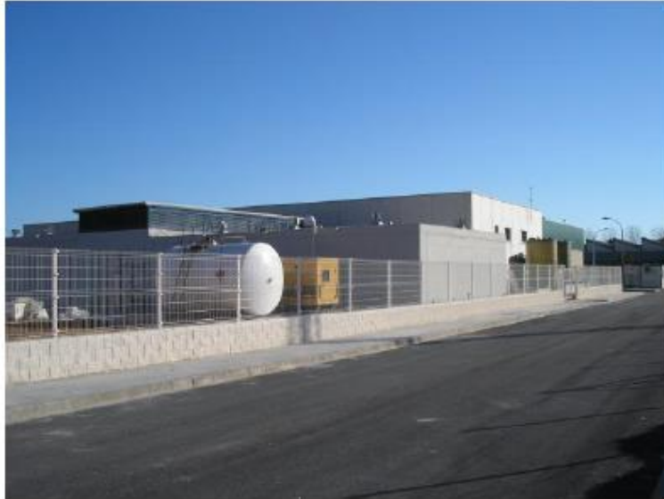
Figure 1: Falconera Water Treatment Plant
