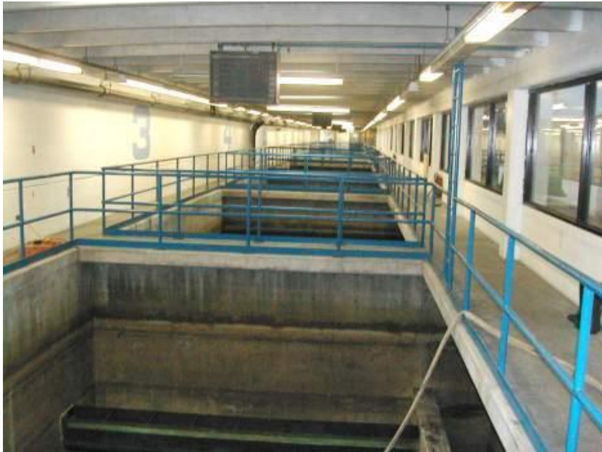
28 MGD (106 MLD) Before
